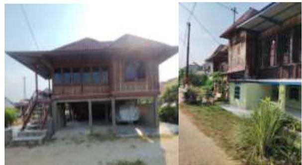
**Image 8.** Hollow Foundation Section (Left) and Foundation Section, which is Used as a Closed Room (Right)
