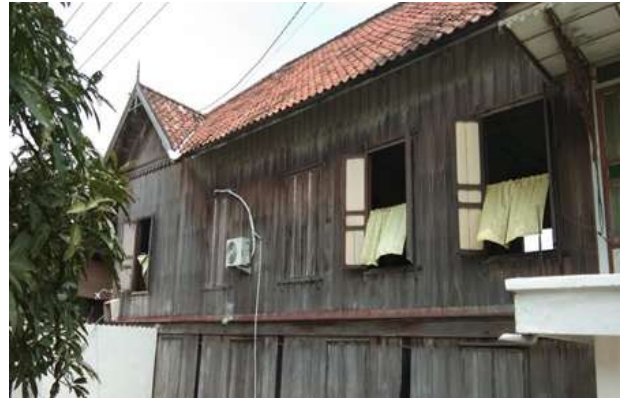
Figure 4. The right exterior view of the stilt house shows its structure, made of ironwood.
