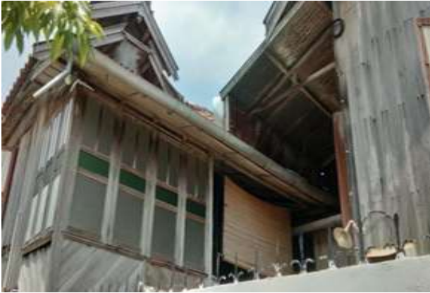
Figure 8. Interior of the corridor between the rooms of the stilt house with wooden floors that are still sturdy after decades Source: Authors, 2024.
