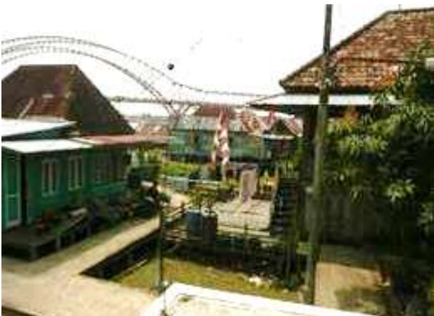
Figure 10. Side view of the Stilt House showing the relationship of the building to the surrounding environment Source: Authors, 2024.
